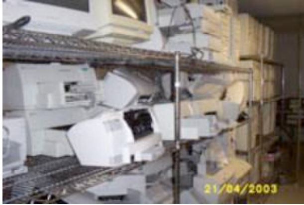
This is the vault where we keep our extra hardware
